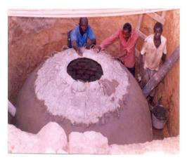
Biogas production in Kayes, Mali. Via this digester, cow dung is used to produce biogas.
