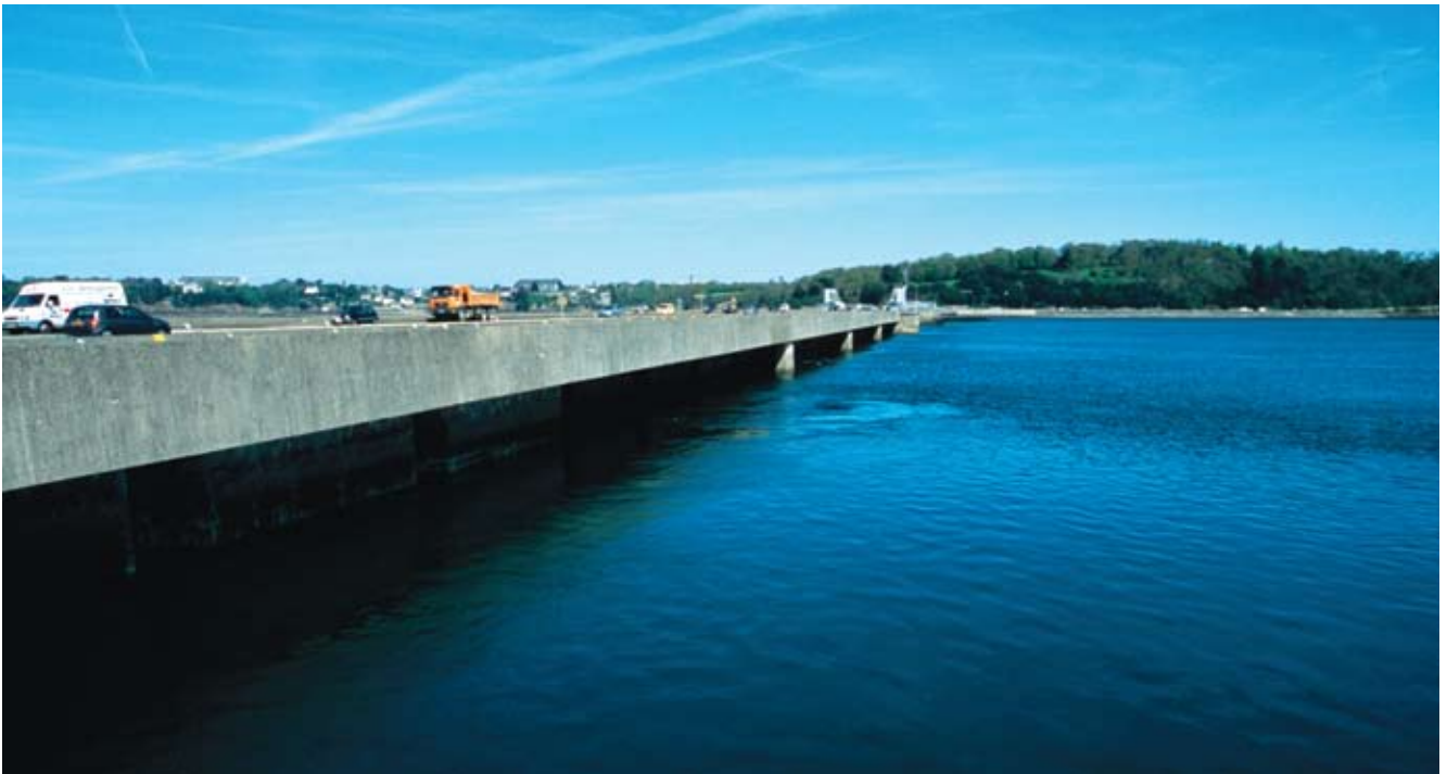
Barrage Plant, Rance Estuary, Brittany, France
