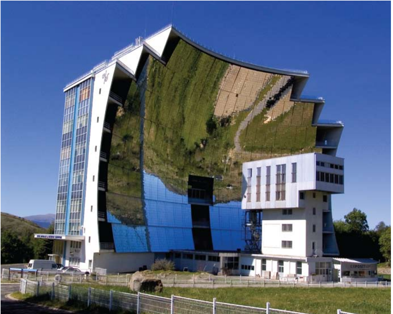
Solar thermal collector, Font-Romeu, France
