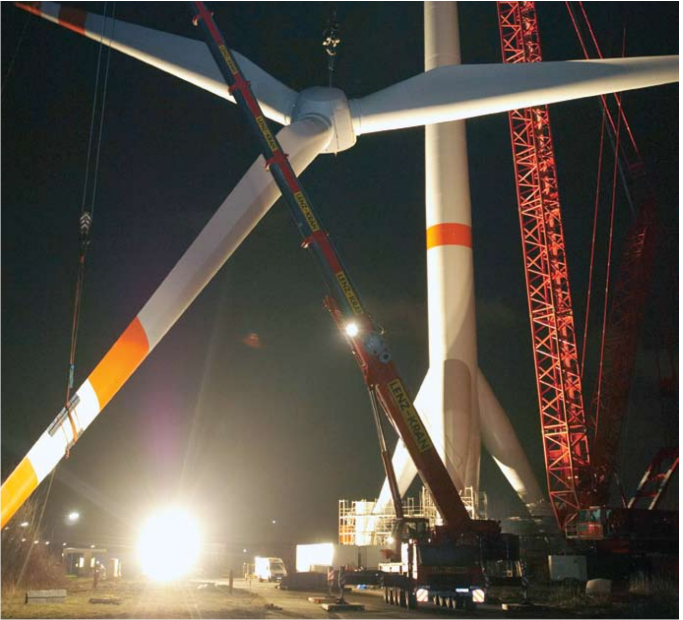
Construction of the Bremen Windfarm
