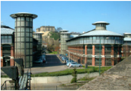
CASE STUDY: CHP (COMMERCIAL, RESIDENTIAL)
